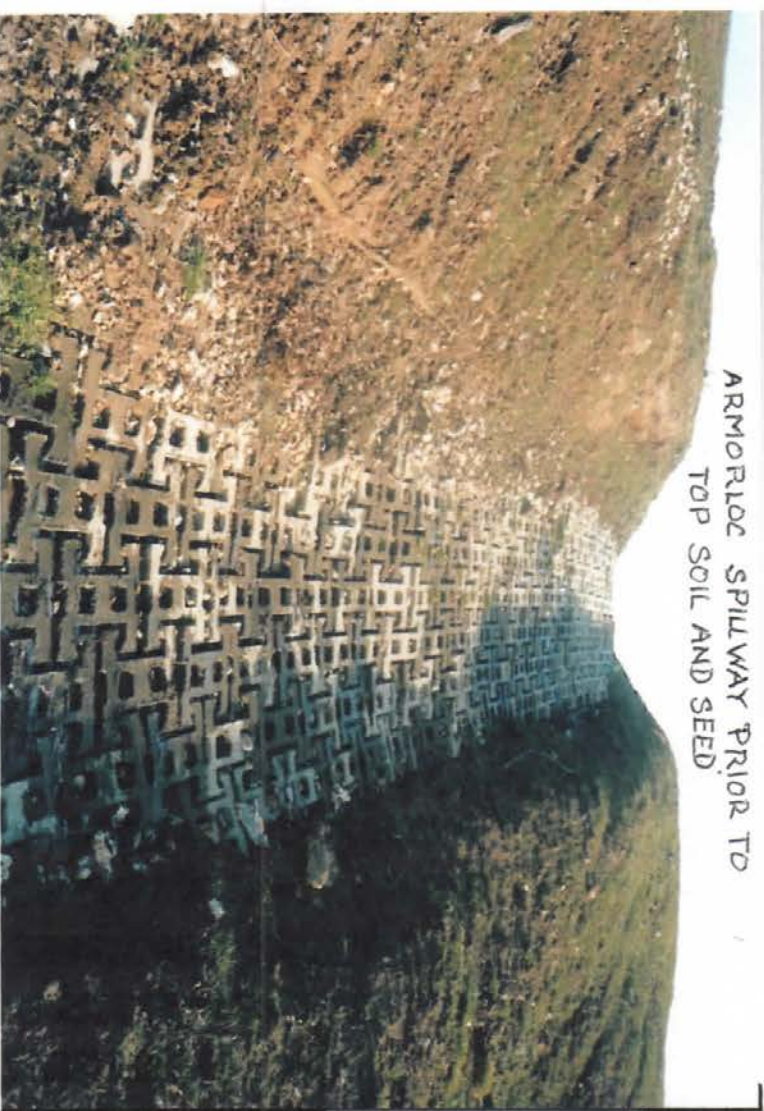
ARMORLOC REVEGETMENT BEING COVERED WITH SOIL
