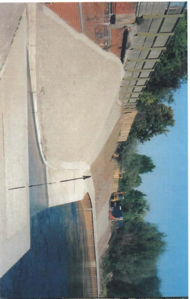
ARMORLOC REVEGETMENT BEING COVERED WITH SOIL
